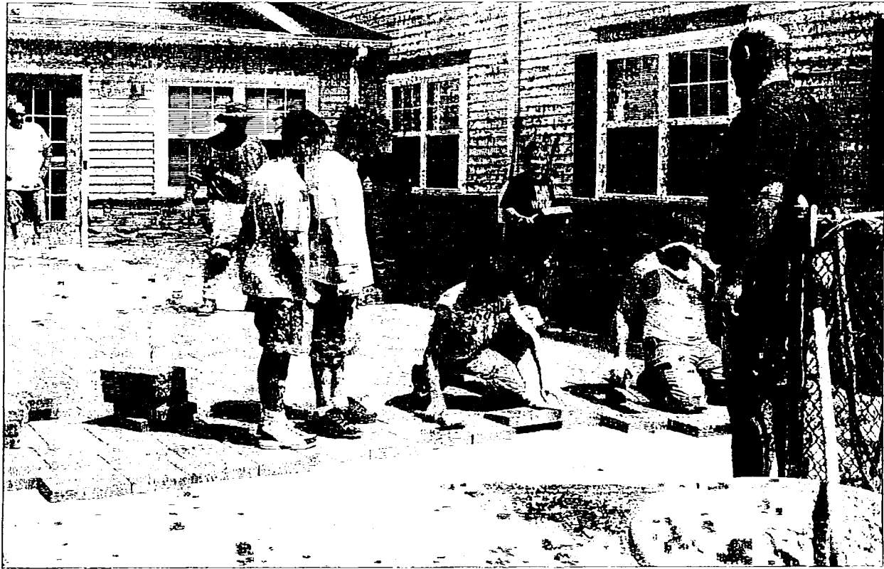
Boy Scouts from Troop 52 of Toms River work on a patio at Dottie's House in Brick. The construction was organized by 13-year-old Kyle Reid (kneeling, center) as his Eagle Scout project. (PHOTO: COURTESY OF KYLE REID)
